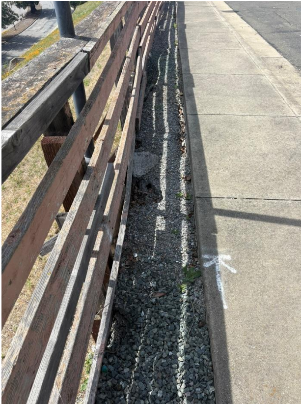
PHOTOS 3 and 4: Site Condition C: Voids in the Gravel Backfill (left) and Current State of Wooden Retaining wall (Right)
